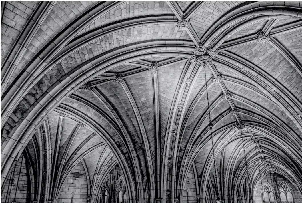
Figure 3. A Vaulted Ceiling 31
