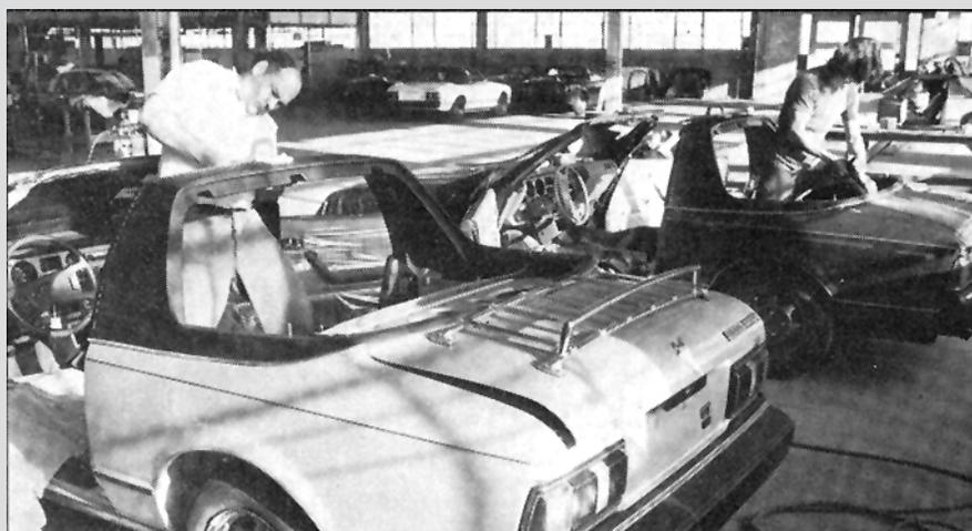
struction techniques. Working with Griffith's part-panel-part-ragtop idea, Deaver devised a combination structural-reinforcement / cosmetic-looker / top attacher made from laminated fiberglass. 'These pieces were created by hand - still are - and entirely covered the raw metal edge, where the steel top once resided. Both the liftoff panel and the cabriolet convertible top were attached to this hoop, mak-
