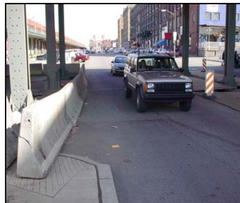
Sidewalk Ending Forcing Pedestrians into Traffic
